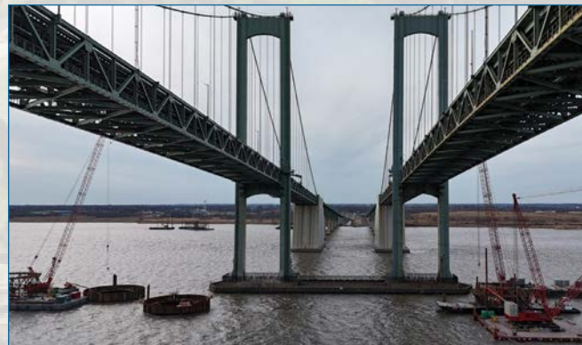
Memorial Bridge “Dolphins” Designed to Stop Ships
